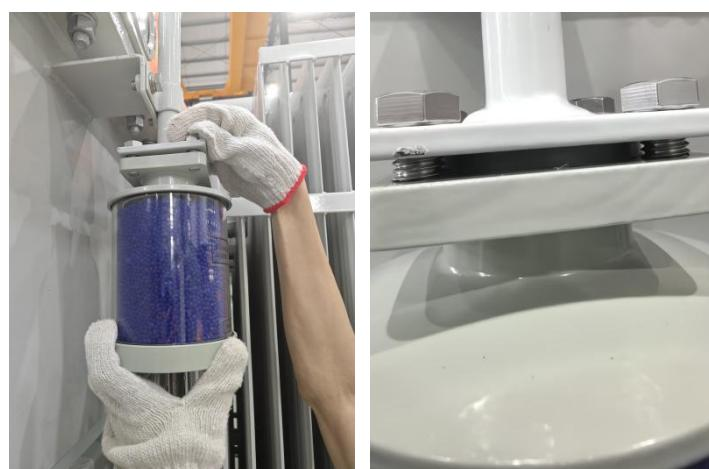
**Step 5:** Remove the oil cup and fill the cup with oil level between the two red lines.
