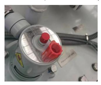
Figure 6-5 pressure relief valve safety cover
