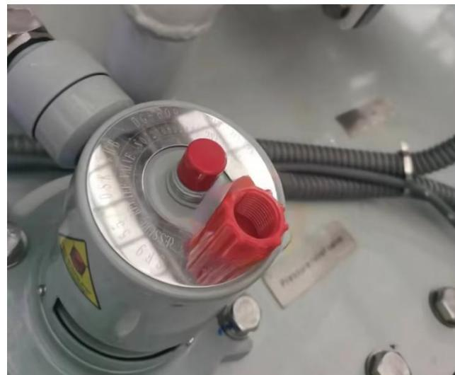
Figure 6-5 pressure relief valve safety cover
