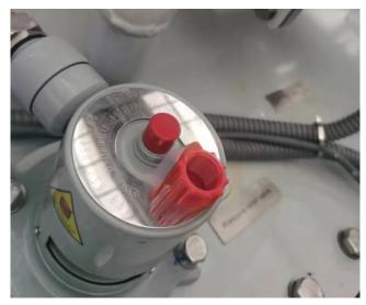
Figure 6-4 pressure relief valve safety cover
