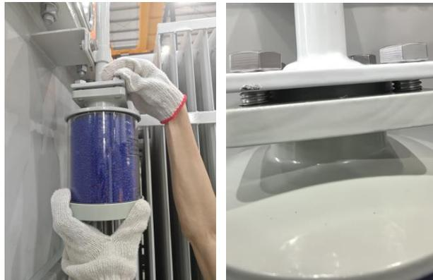
5) Remove the oil cup and fill the cup with oil level between the two red lines.
