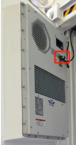
2) Remove a circle of fixing screws around the air conditioner and remove the air conditioner (M5 hexagon socket bolts)
